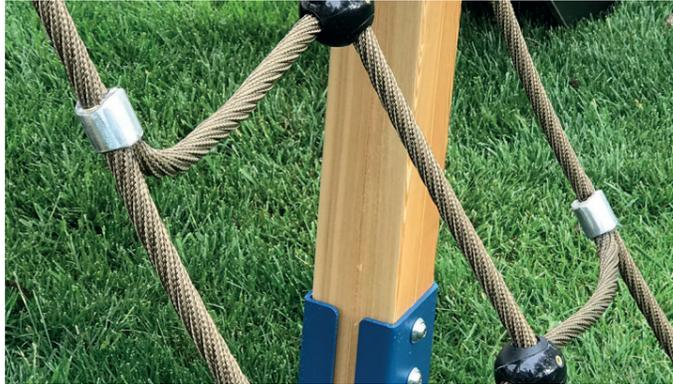
**CMRope™ is formed by 6 strands of galvanized wires and a core either steel or fiber. Each strand is tightly braided with Polyester which is adhered to galvanized wires with a patented method to create a solid surface where polyester meets with wires. So extra protection is achieved against friction and vandalism. Surface is extremely abrasion and UV resistant also fire retardant.**
