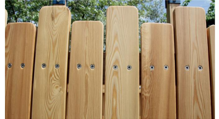
**The yellow pine or black pine, used as first class and oven-dried, is much more resistant to environment and weather conditions compared to white pine. Humidity rate is 10-12%. There is no decayed or joined knurl. It is suitable for all kinds of wooden application and coloring.**
