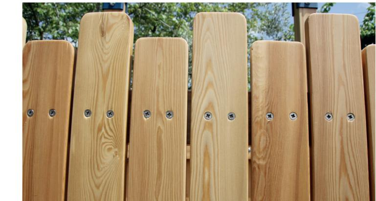
**The yellow pine or black pine, used as first class and oven-dried, is much more resistant to environment and weather conditions compared to white pine. Humidity rate is 10-12%. There is no decayed or joined knurl. It is suitable for all kinds of wooden application and coloring.**
