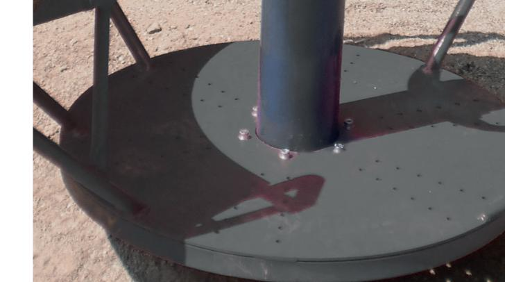
**Platforms are made of plastic-coated steel sheets which are decorated with drainage and holes. Plastic coating provides further protection against falls and weather conditions.**
