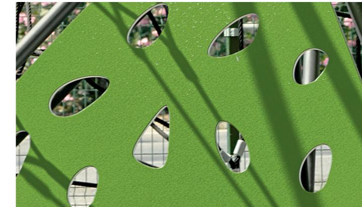
**High quality panels made of HDPE panels are milled to provide a smooth, gently rounded edge. The thickness of the panels varies according to its purpose for floors, roofs, and walls.**
