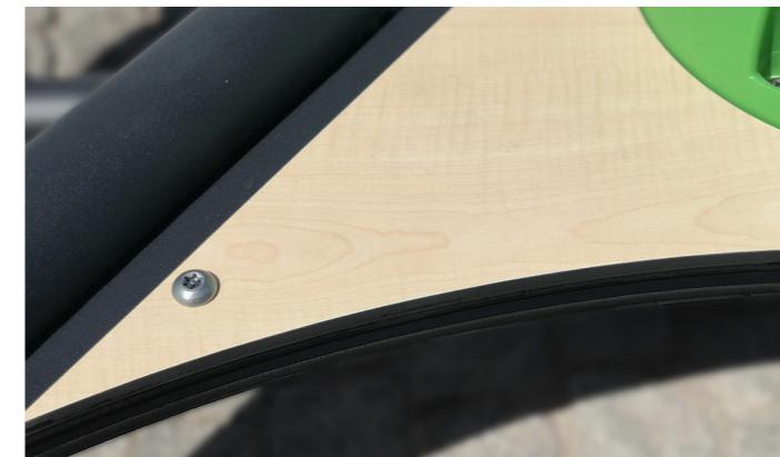
**Exercise panels are made of 12mm HPL panels with high UV resistant and fire retardant. To increase exercise comfort, HPL minimize the generation of electrostatic charge by contact-separation or rubbing with another material.**
